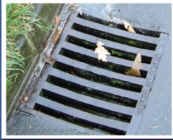
Surface water road drain.
