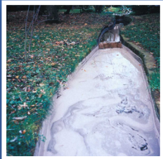
Cement grout entering a stream which resulted in the death of a number of Carp.
