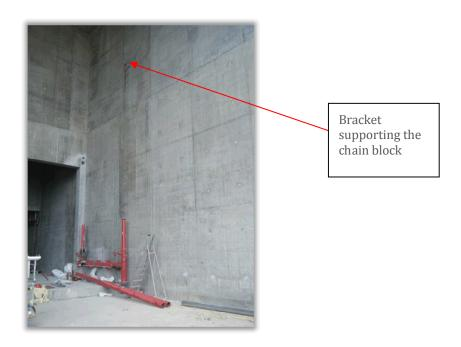
The investigation identified that the means by which the pipe had been slung (i.e. attached) to a chain block being used to carry out the lifting of the pipe was inappropriate. As the pipe was lifted the sling slipped off the pipe causing it to fall to the ground. As the employee tried to run clear he tripped over a change in floor level and fell. The pipe landed on his leg before it came to rest on the ground.
