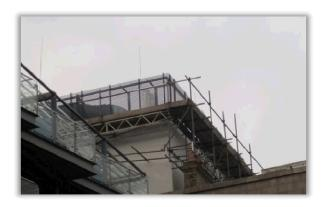
The Inspectorate contacted the scaffold contractor who had erected this scaffold, following concerns made about the manner in which it had been supported on a chimney stack.
