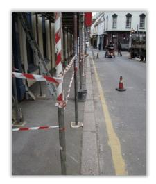
Work being carried out on the roof of a property in St Helier resulted in a complaint being made over material falling into the roadway. In addition to this concern, the scaffold contractor was advised about the need to improve protection for the public during the erection of an uncompleted section of the scaffold.
