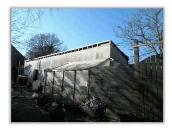
As a result of no edge protection being provided to the roof of this building, which was being re-roofed, work was stopped.
