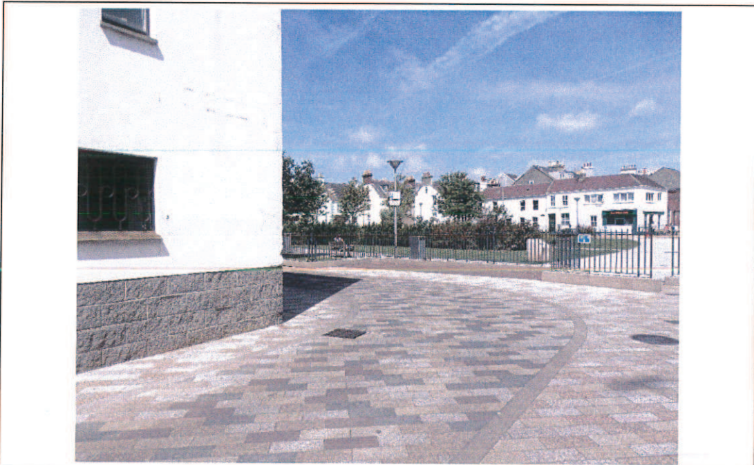
D13 The delineation between the carriageway and footway (photograph taken by A Luck on 8 th July 2016)
