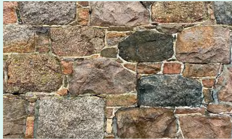
Local natural stone cladding used to walling.
