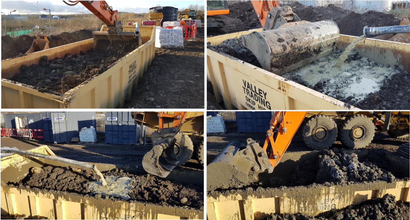
Figure 27 – Ex-situ E-Clay Stabilisation Process
