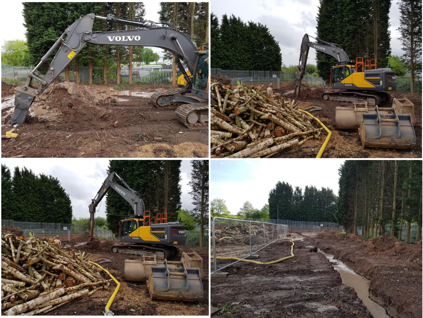
Figure 19 – E-Clay PRB Installation – Trenching Methodology
