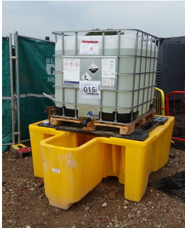
Figure 34 – Typical Chemical Containment Bund
