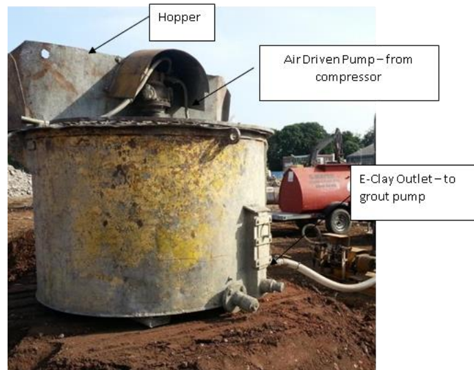
Figure 28 - Grout Mixer used for the Production of E-Clay Slurry
