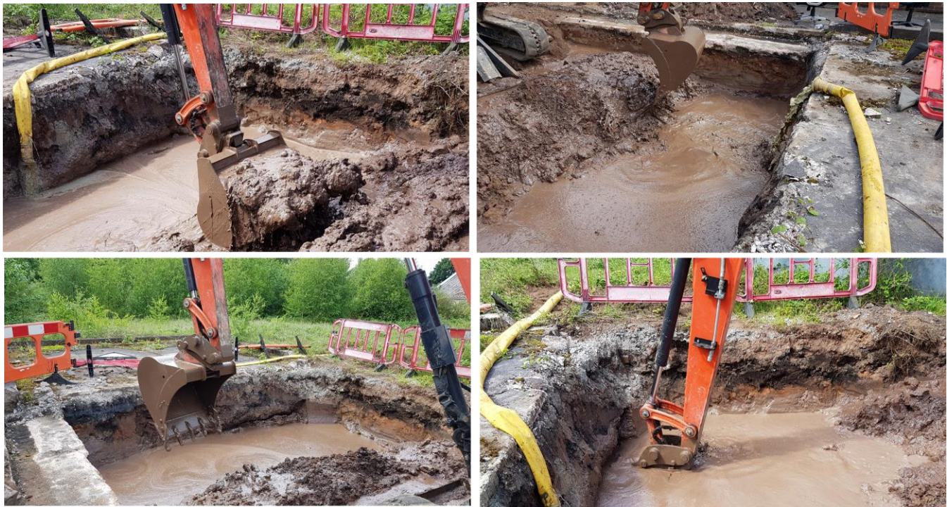
Figure 24 – In-situ E-Clay Stabilisation Process
