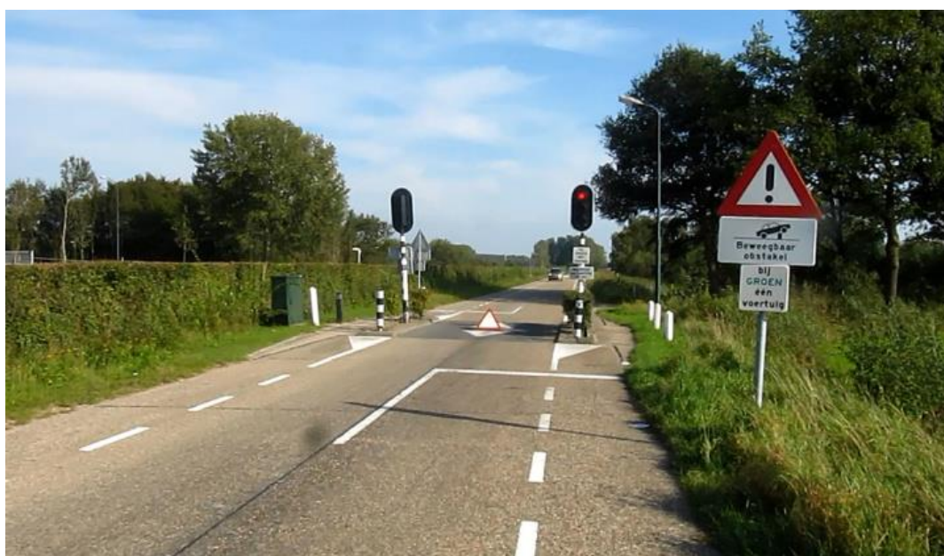
Figure 0-36: Rising bollards are used on larger rural roads in The Netherlands where some local access is required
