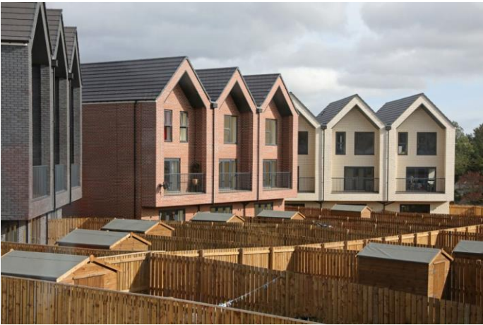
Image 12 - Gateshead Innovation Village (Credits: Constructing Excellence)
