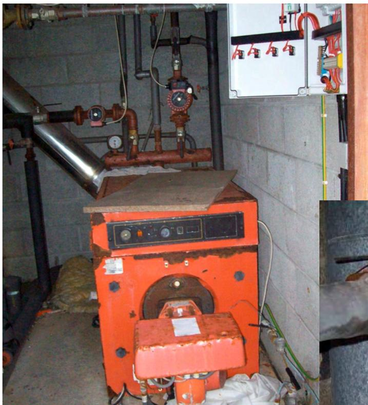
It appears that the central heating system was fuelled by oil. The site oil tank is located at the NW corner of the site. Therefore it is assumed that there is an underground oil distribution network to feed each boilers.
