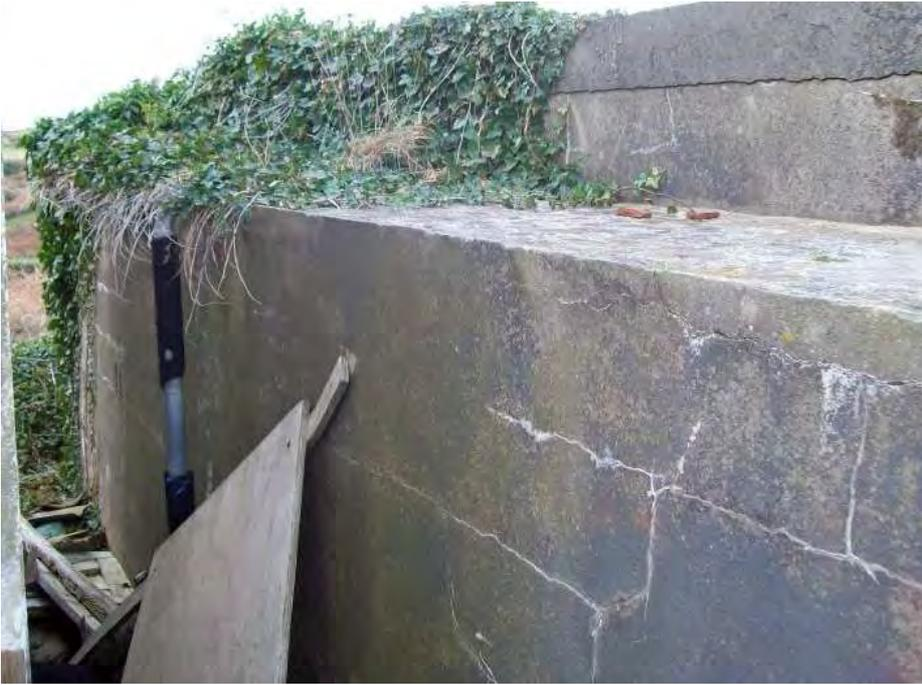
To the south of the tennis court there is the water treatment tank. This consists of a large rectangular concrete structure, which extends approximately 1.2m above ground.
