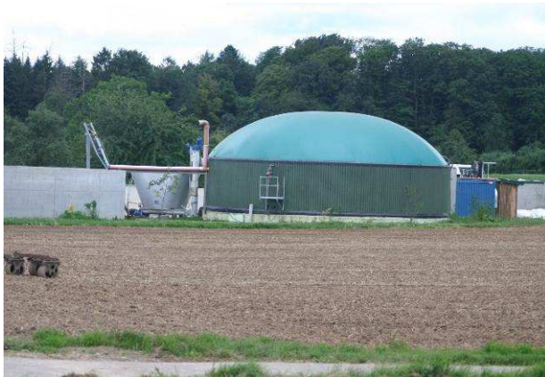
Figure 11 Gas Holder Constructed on the Top of Digester Vessel
