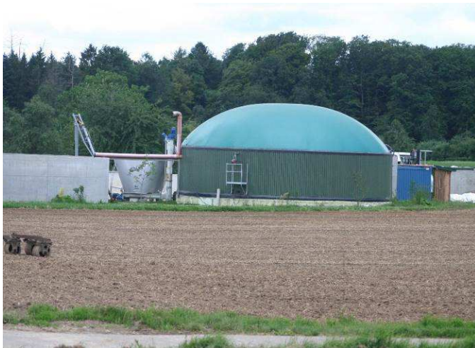
Figure 6 Wet AD Digester Vessel
