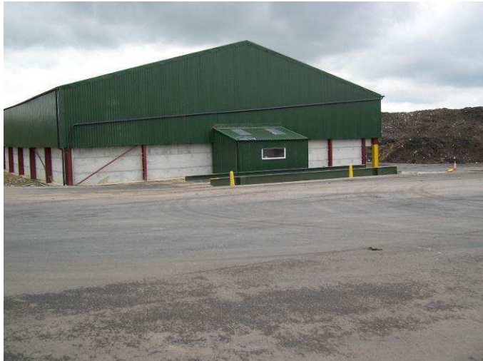
Figure 5 Full size vehicle weighbridge, with reception hall
