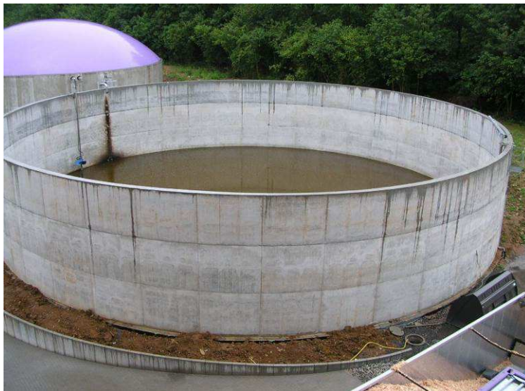
Figure 7 Covered and uncovered circular store for digestate storage
