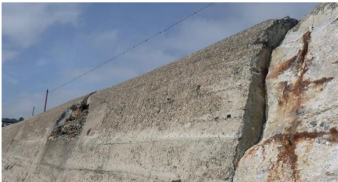
Figure 2-2 Photograph showing current condition of seawall
