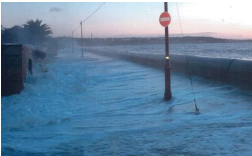
Figure 3-3 Photograph showing overtopping of seawall
