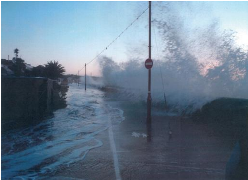
Figure 3-3 Photograph showing overtopping of seawall
