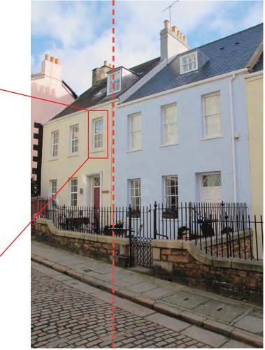
Example historic window Example historic glass detail retained replaced with inappropriate UPVC units
