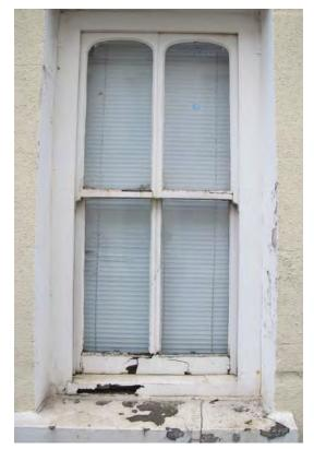
Example of decay to Timber Sash Window through poor maintenance
