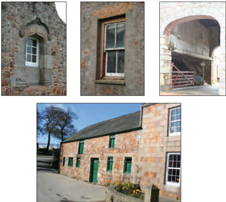
Figure 19. Materials and Detail. A characteristic late medieval Jersey French ogee-headed arch (top left) and a late 19th century example of a sash window with plate-glass panes used on a working building (top middle). View into an through-way at La Falaise, St John, showing what is now a rare surviving example of timber internal partitioning to working buildings (top right). The distinction between domestic and working buildings is clear in this linear range (bottom), with the house using ashlar stonework in contrast to the coursed rubble on the working buildings, and the rare survival of plank doors and shuttered openings to adjust the ventilation of the cattle housing and loft.
