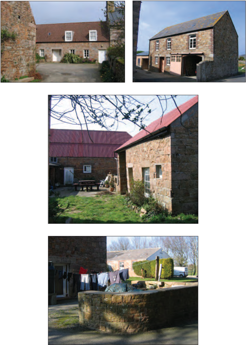
Figure 25. Farm buildings in Jersey (see glossary for more examples). The cider house (top left, with its wider door) and stable in the same U-shaped farmyard as Figure 23 (below). A combination building (top right): sliding doors as here were widely introduced from the later 19th century. A detached bakehouse (middle) and a manure tank marked by its curved wall and pump (bottom).
