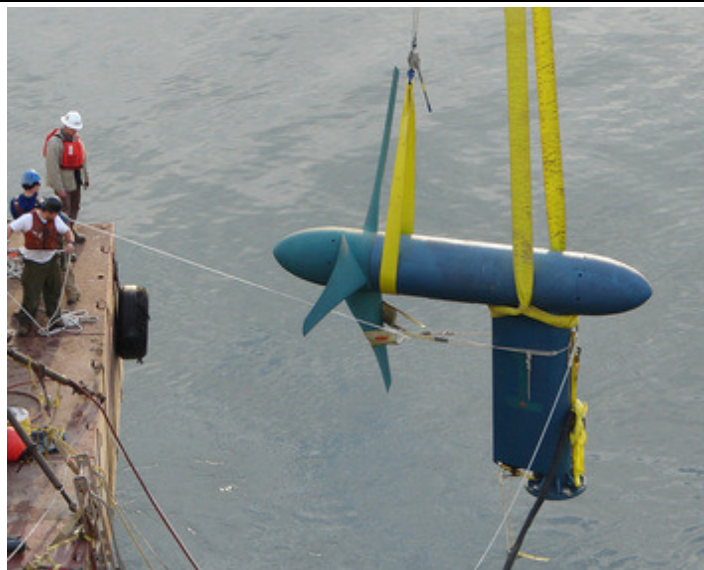
Figure 10, Verdant's Gen 5 turbine during installation in New York
