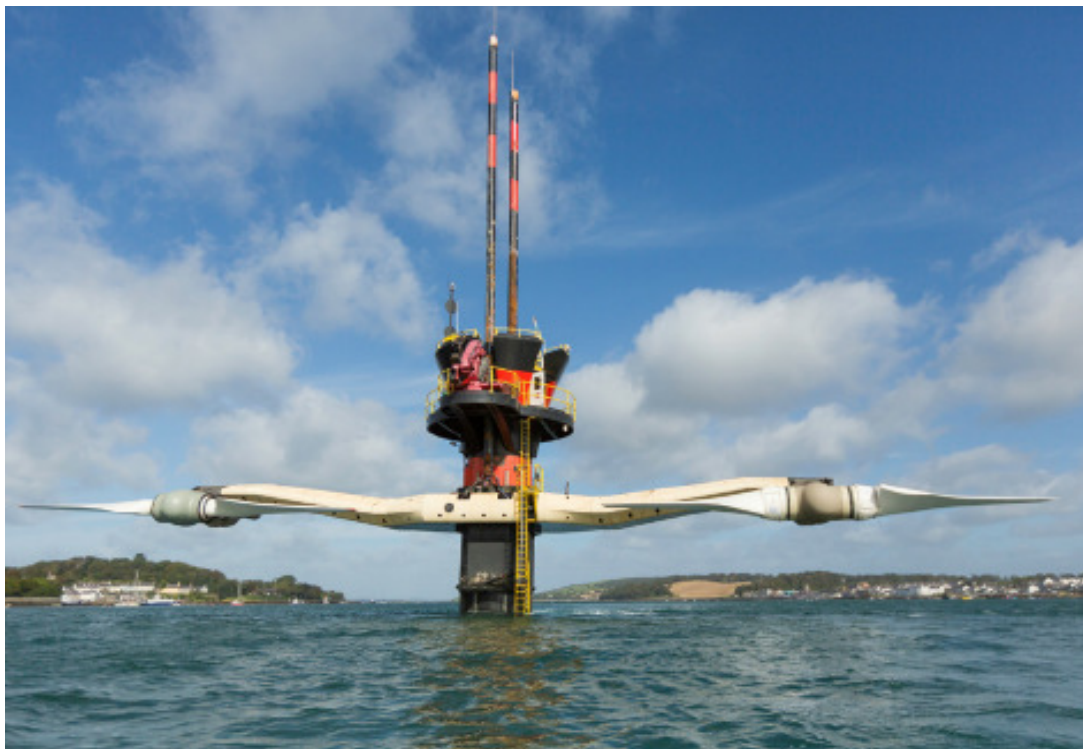
Figure 3, MCT's 1.2MW Seagen turbine in Strangford Loch
