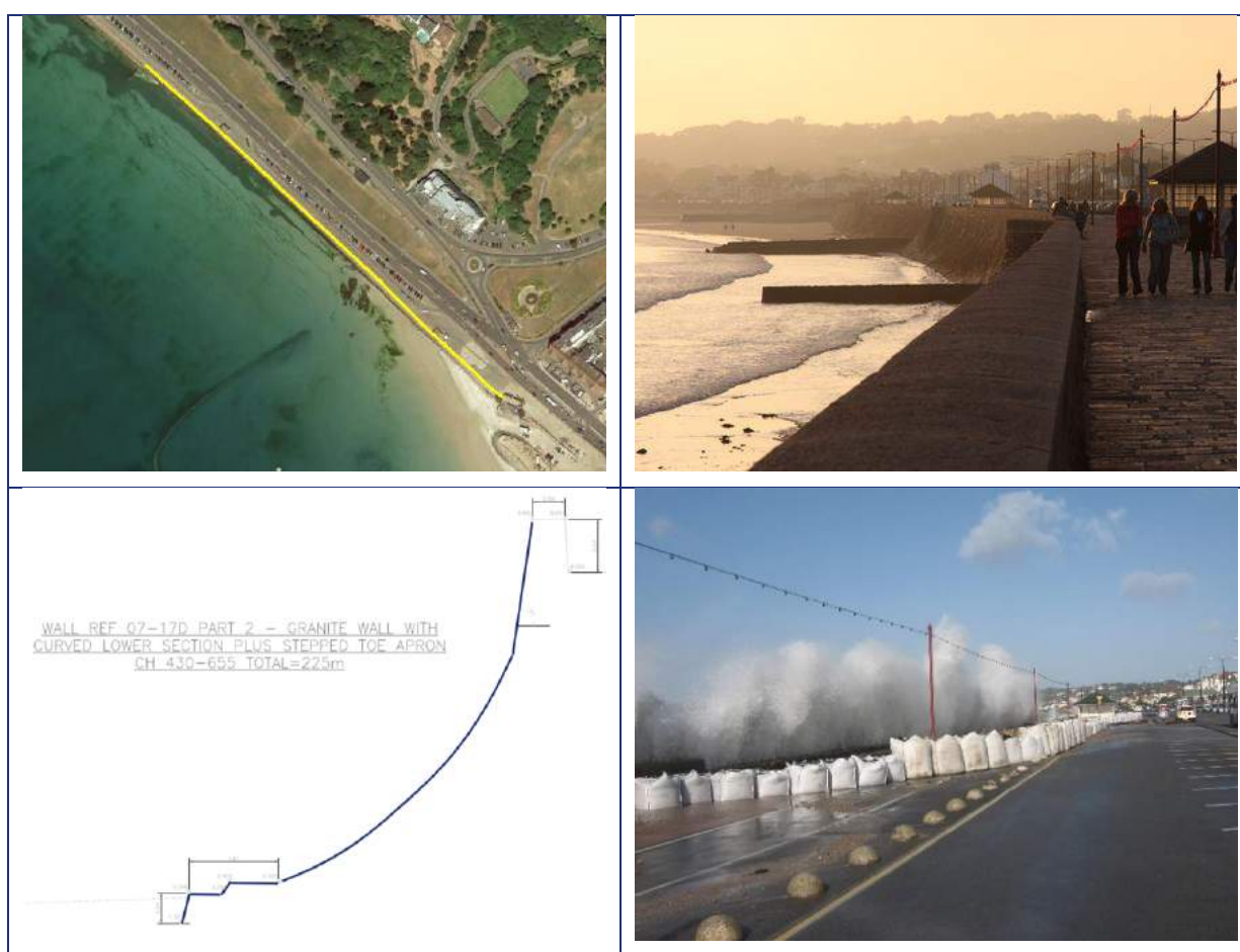
Figure 6-1: Structure and overtopping evidence at Structure 1: Victoria Avenue seawall
