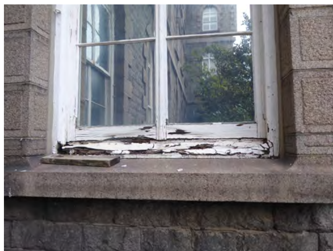
Timber window in front façade showing signs of decay
