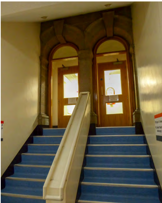
Former window openings at second-floor level in north of the Granite Block adapted to form door openings
