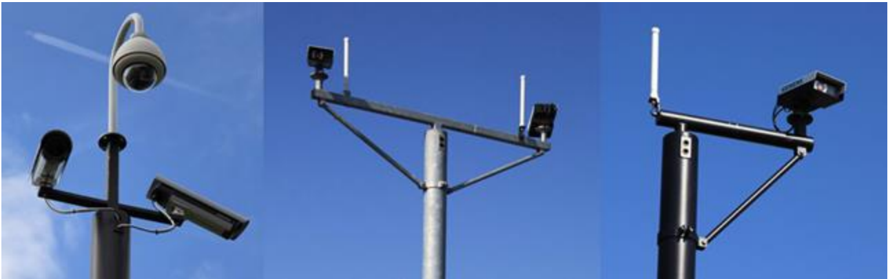
Figure 1: Pole mounted CCTV arrangements
