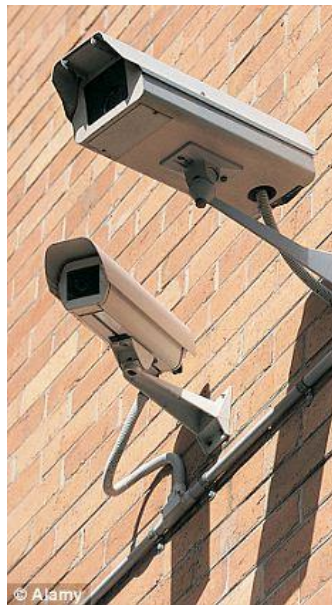
Figure 2 – Building mounted CCTV arrangements
