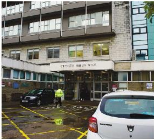
■ The current hospital is deteriorating and requires millions to be spent on maintenance
