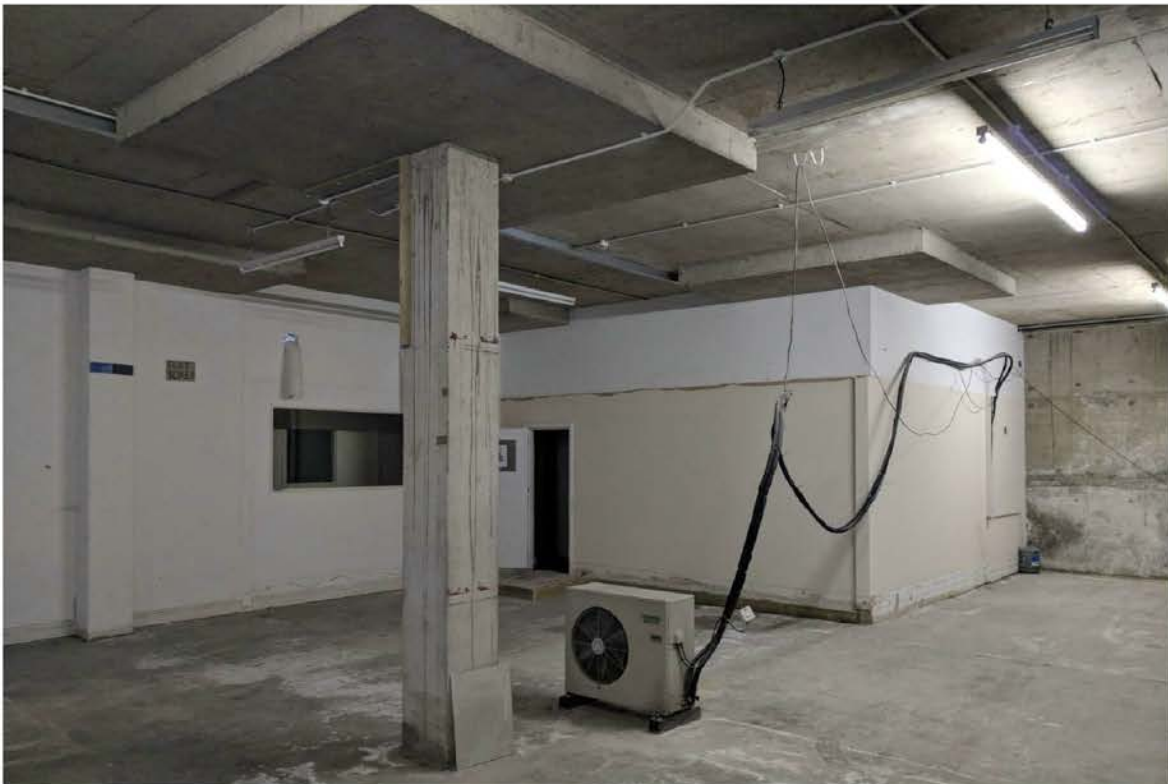
View of Existing Office Area
