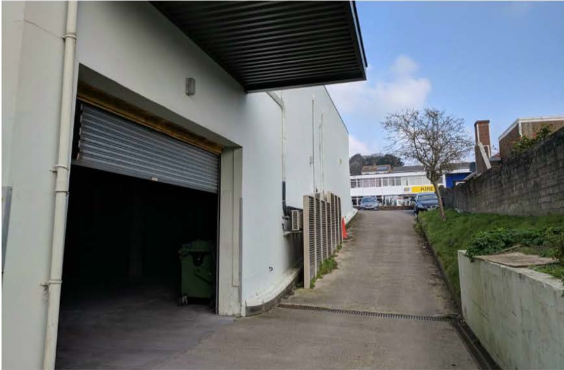
Existing Access Ramp looking North
