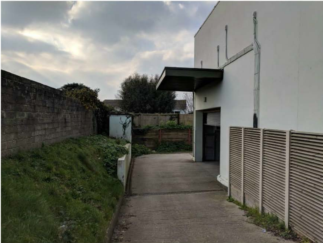
Existing Access Ramp looking South
