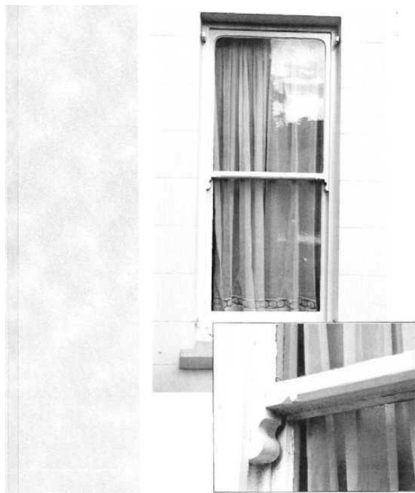
Single-pane sash with chamfered meeting rail, diamond chamfer stop and decorative horns, St Helier
