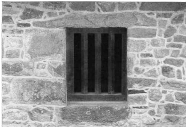
Chamfered timber mullions, designed to allow the infiltration of as much light as possible, Hamptonne, St Lawrence
