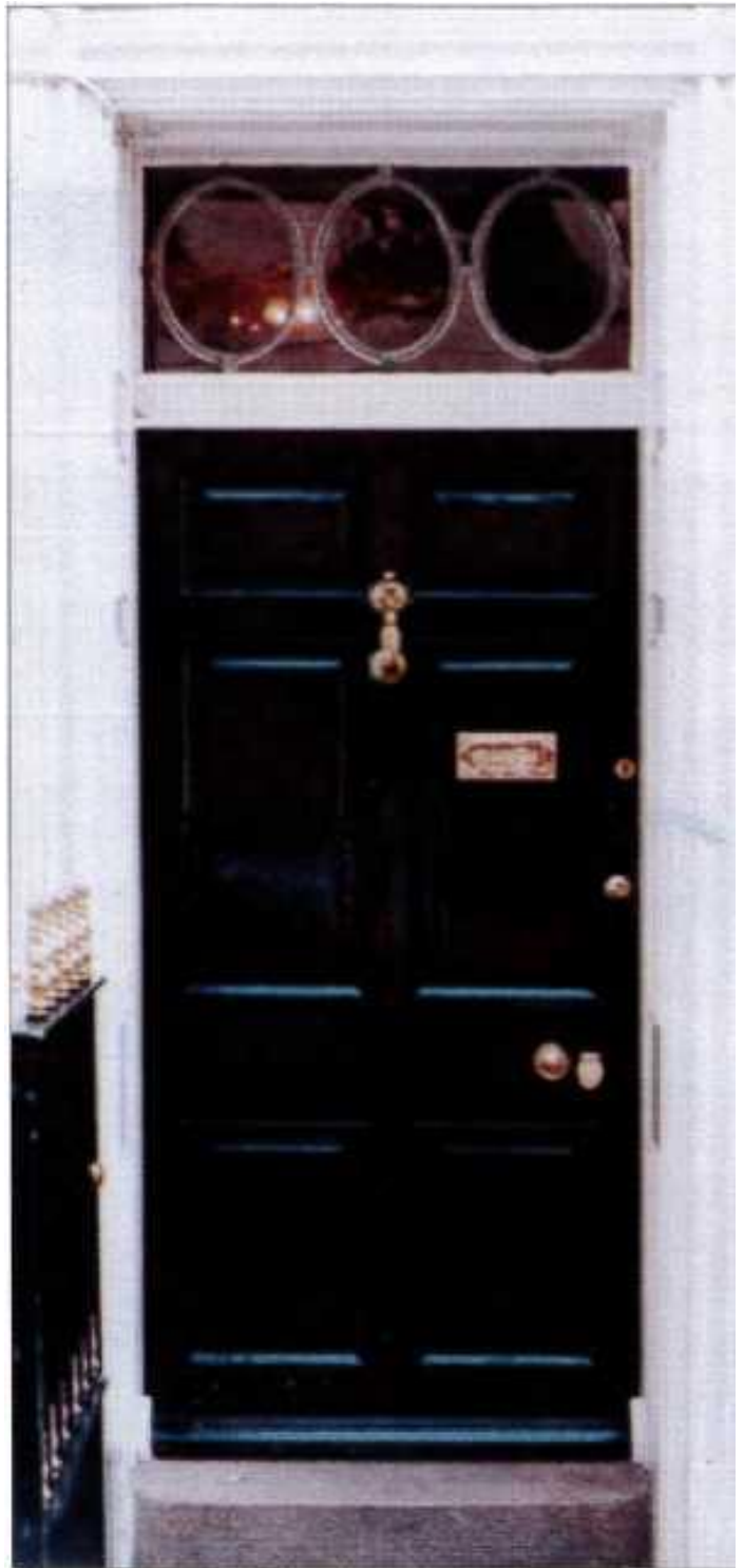
Six raised-and-fielded panel door, with fanlight over, St Helier.
