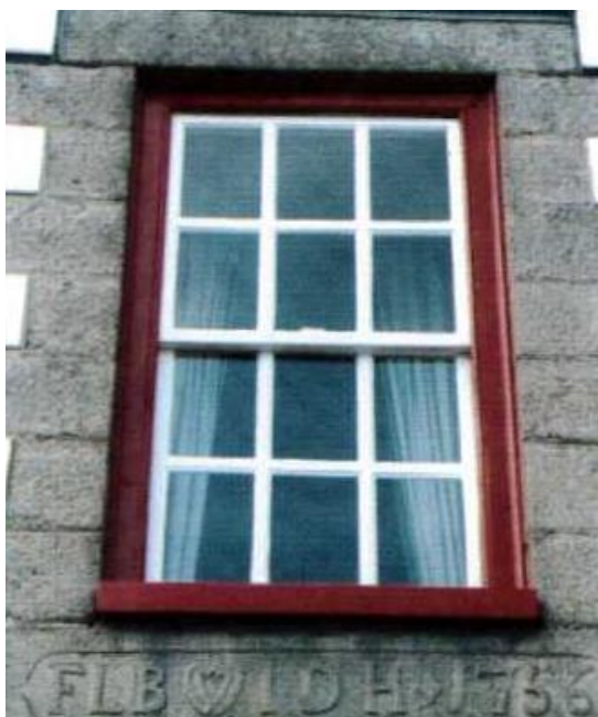
One of the earliest sash windows in St Helier at Hue Street - the building is dated 1756. Note the very wide and flat glazing bars, typical of this early style.
