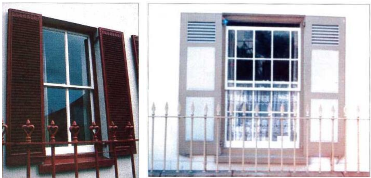
Two types of shutter found in St Helier – a louvred shutter with "keyhole" detail and a solid shutter. Note how the colours have been picked out to match the sash window boxes, cills and railings.
