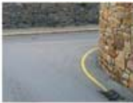
BASIC UTILITARIAN concrete footways, asphalt carriageway, stone kerbs
