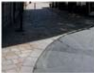
HIGH QUALITY UTILITARIAN stone pedestrian surfaces, asphalt carriageways, stone kerbs
