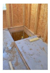
As well as managing the presence of these openings in floors, work to the walls of the stairwell also poses a particular problem for contractors in terms of safe access. It is vital that the sequence of works is carefully considered and the system of work used is properly planned. Unfortunately, the arrangement shown in the photograph below is all too common. This is entirely unacceptable and action will be taken where this type of practice is observed.
