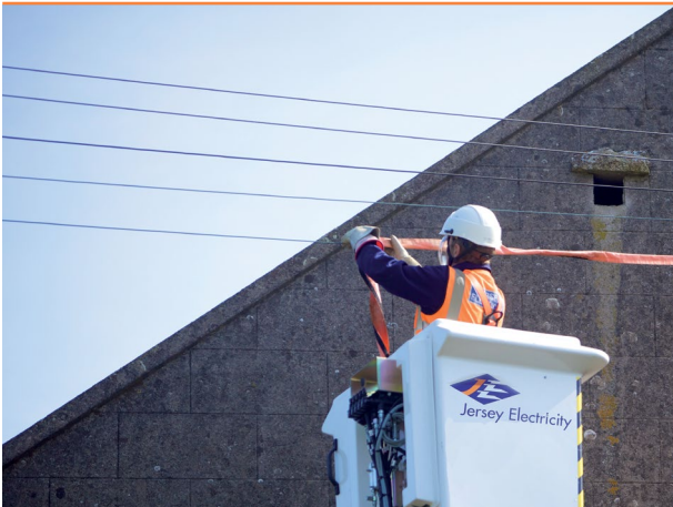
Our engineers sleeve overhead lines for your protection
