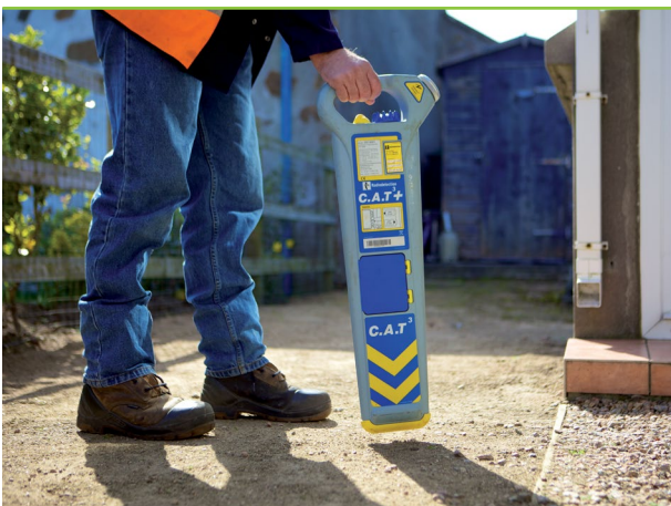
Checking the precise location of our underground cables
