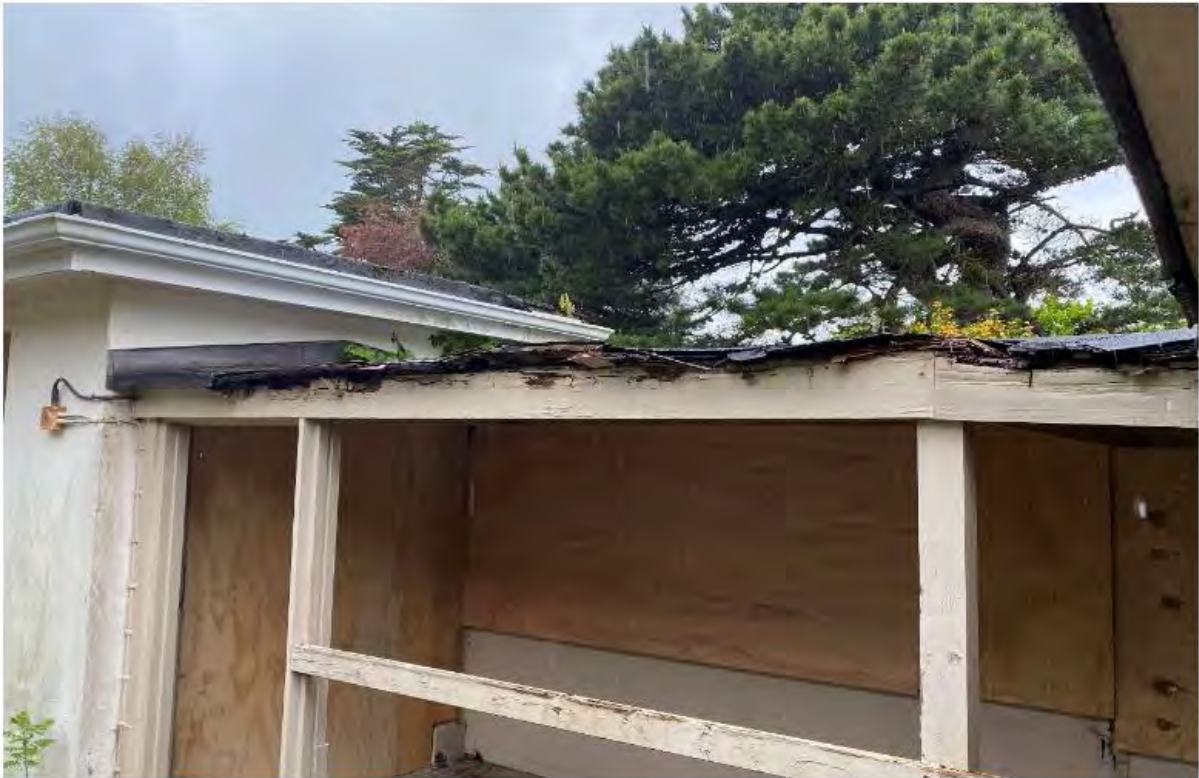
Typical Roof Edge Detail Showing Timber Deterioration
