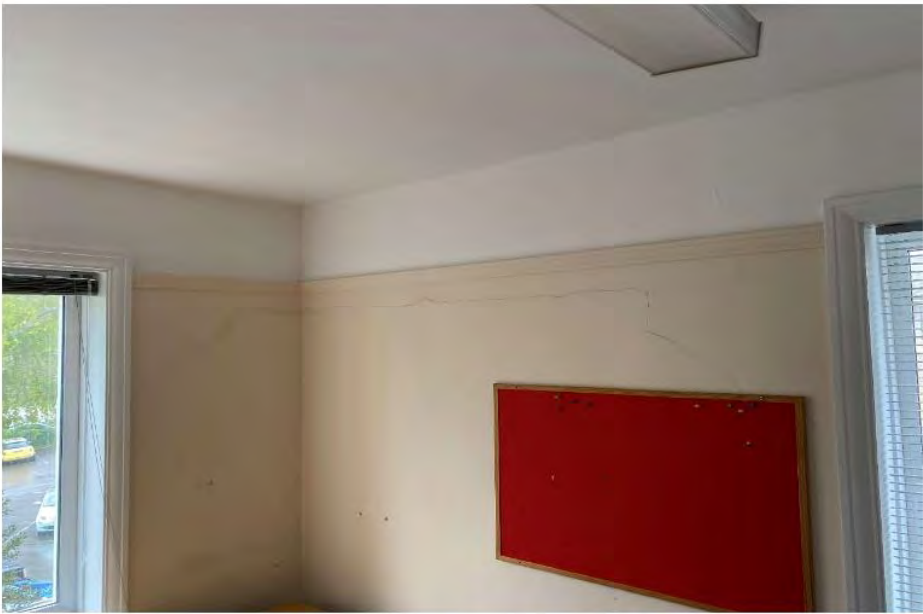
Cracking at Second Floor Level
