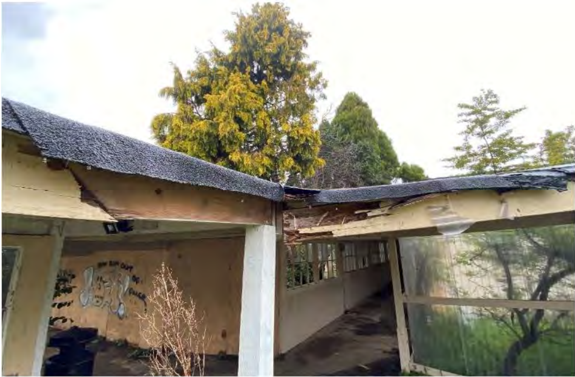
Timber Defects to Central Walkway Junction
