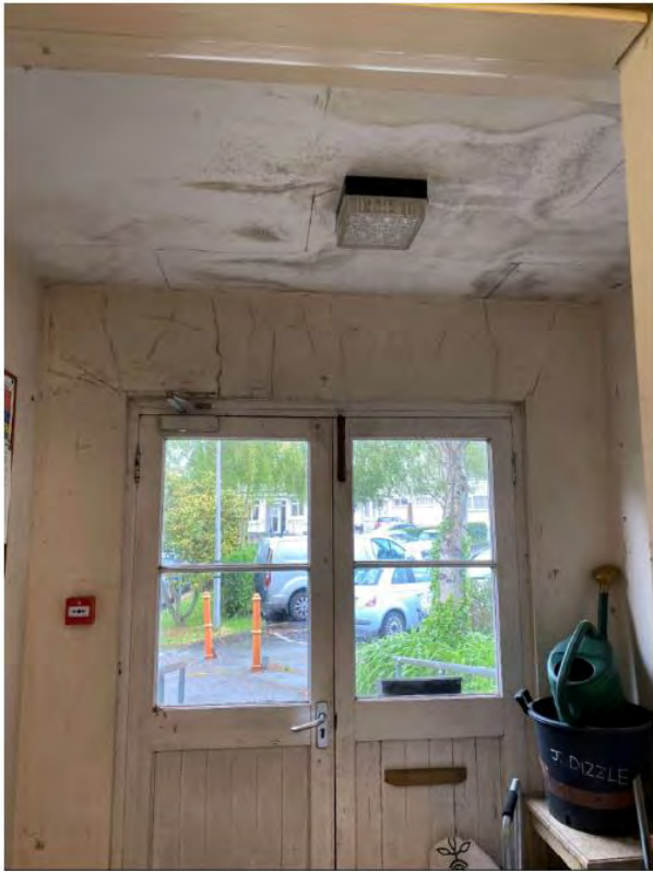
Internal Cracking Over Front Entrance
