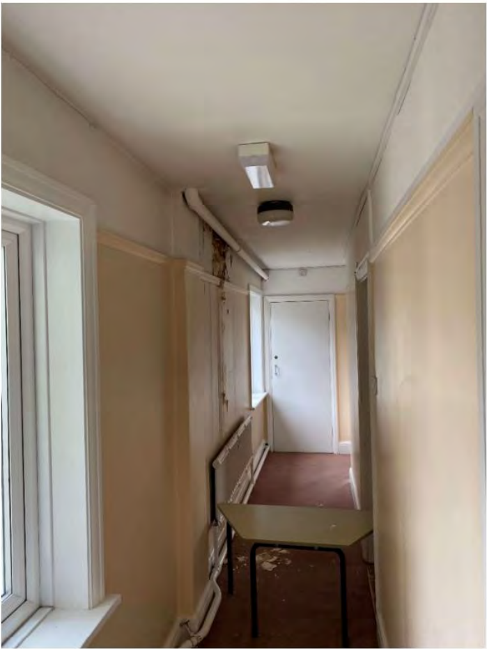
Second Floor Corridor Showing Water Ingress From Roof
