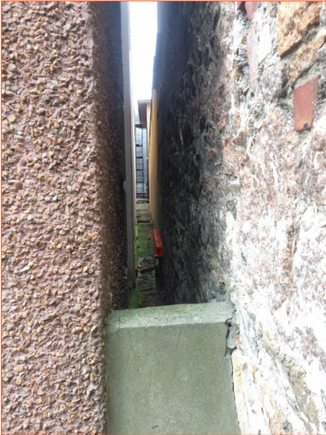
Photo 23 – Showing props between retaining wall and MSCP and unidentified underground structure (highlighted in red) as part of building forming the retaining wall.
