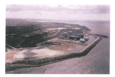
The Flamanville nuclear power plant (CNPE) is situated on Flamanville municipality land, on the coast, in the department of La Manche (50), 21 km south-west of Cherbourg. Designed from the outset to accommodate four nuclear production units, it currently comprises two identical 1300 MWe nuclear units which are pressurized water type reactors and two predeveloped platforms which can host two new units as the aerial photo on the left shows.
