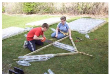
Screw the triangular gables to the posts and include a top beam and vertical supports (from the top of the gables to the top of the front and back panels). The sloping sides of the roof can be made out of similar panels as the walls. These can then be screwed onto
