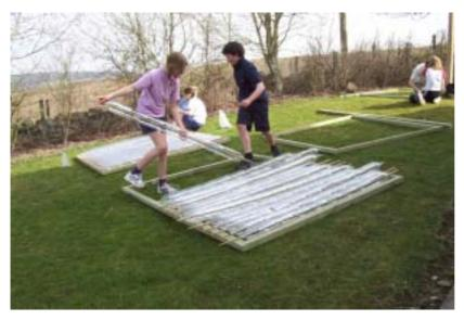
Place the bottles and canes onto the frames to be attached at the top and bottom of the frame.
