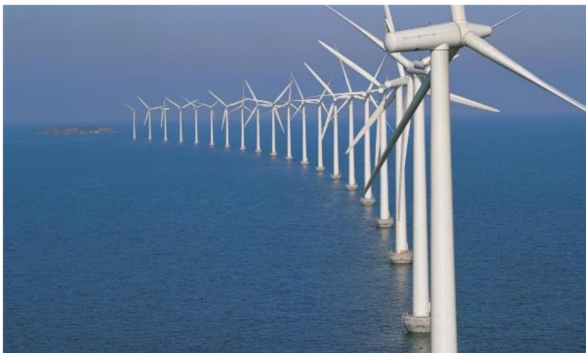
Figure 7-19, The unique shape of the community owned, 40MW Middelgrunden offshore wind farm.
