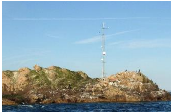
Figure 6-7, Mast on Les Ecrehous – similar to that on Les Minquiers
