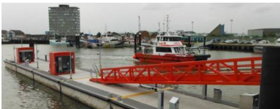
Figure 7-18: Crew Transfer Pontoon for Humber Gateway [Source: Marine Designs Ltd]
