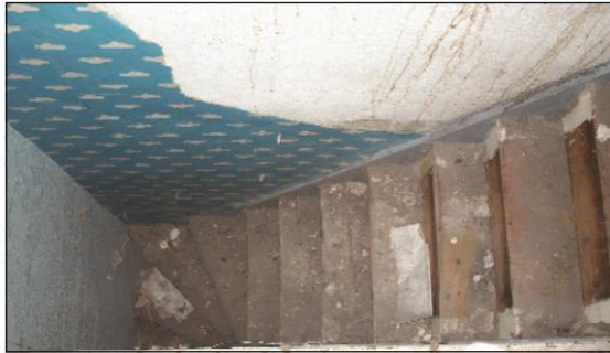
View of stairs from landing
