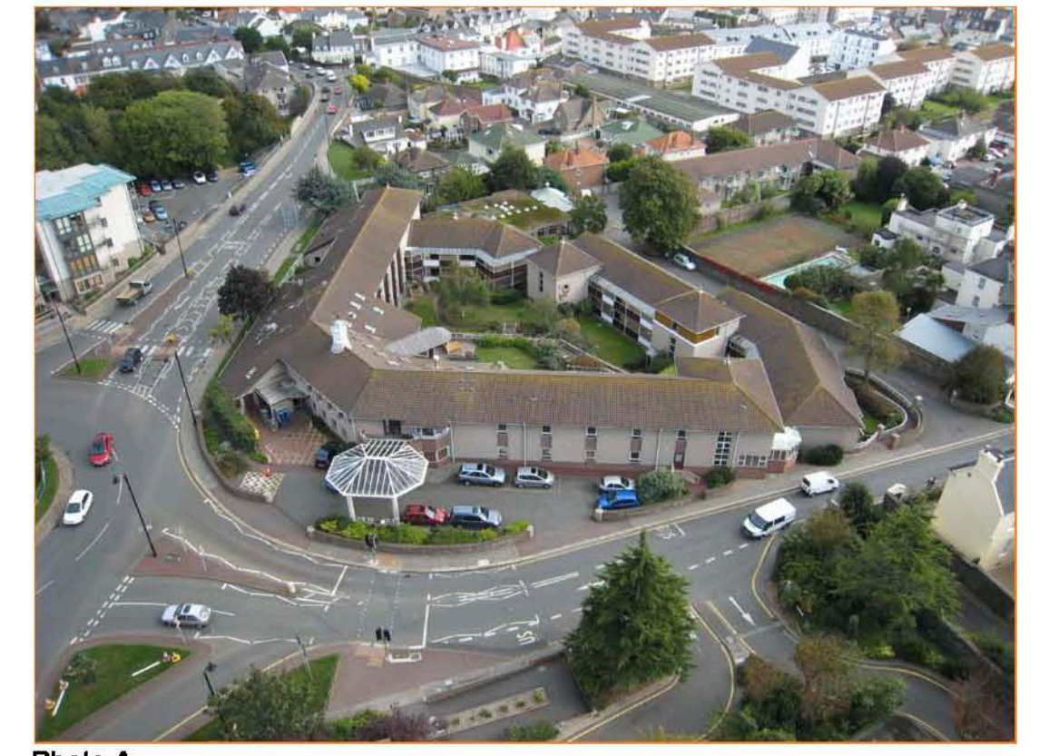
Photo A Aerial photo, in the location of the proposed shelter
