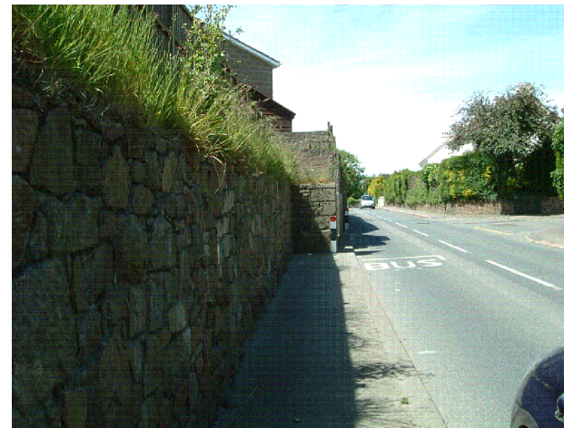
Photo A - View Looking West along Rue a Don
