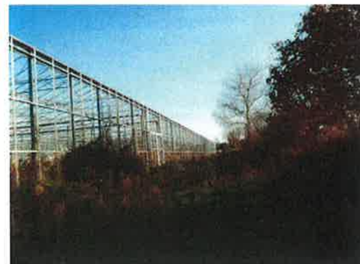
View of southern boundary, looking east
