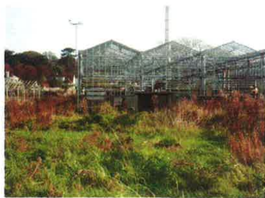
View of southern greenhouse, looking east.
