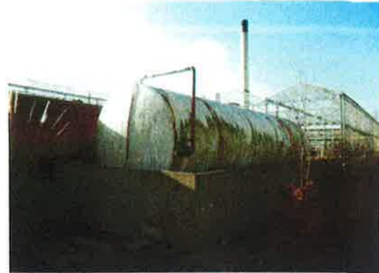
Tank area by southern greenhouse. shows tank within a concrete bunded structure.
