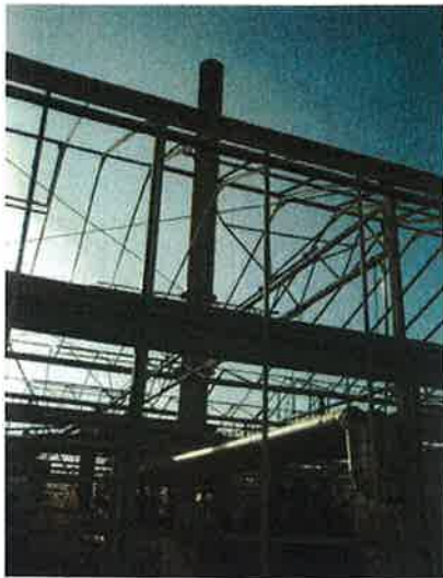
Chimney/flue attached to boiler
