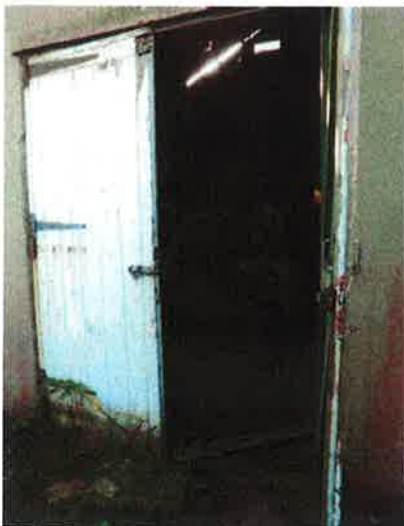
Concrete building by northern greenhouse with two boilers inside.
