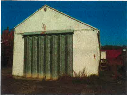
Boarded up concrete building to the north west
