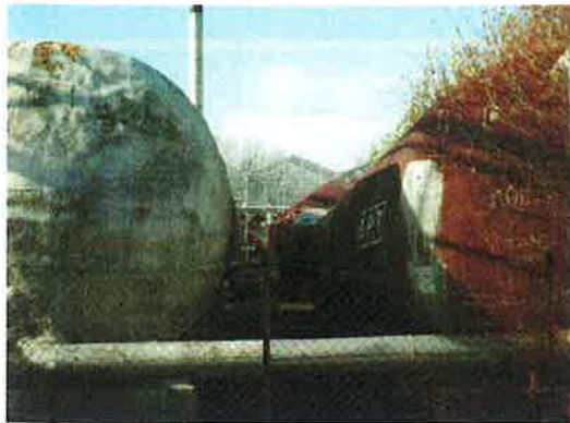
Looking west at tank area, showing misshapen tank wagon on right
