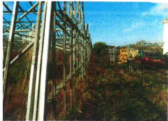
View looking west along northern site boundary with residential properties to the right
