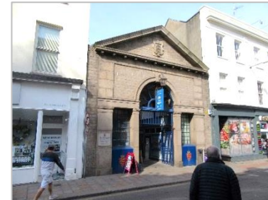
Poor external impact
