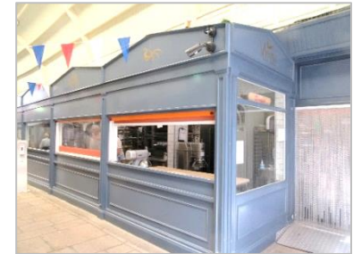
Well maintained external fascia
