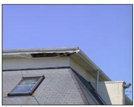
photo 8 Missing soffit boards
