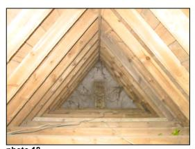
photo 18 Roof interior above ceiling boards.
