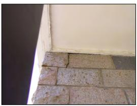
photo 10Missing pointing and loose blockwork.
