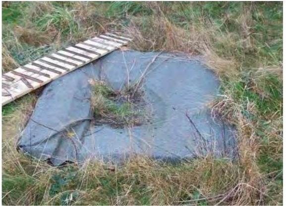
To the east of the sub-station there is wood(rotten) /felt covered service trench. The trench is breeze block lined. It was most likely covered by something more durable when the camp was still working. Permanent access to the pipework must have been needed within this area.
