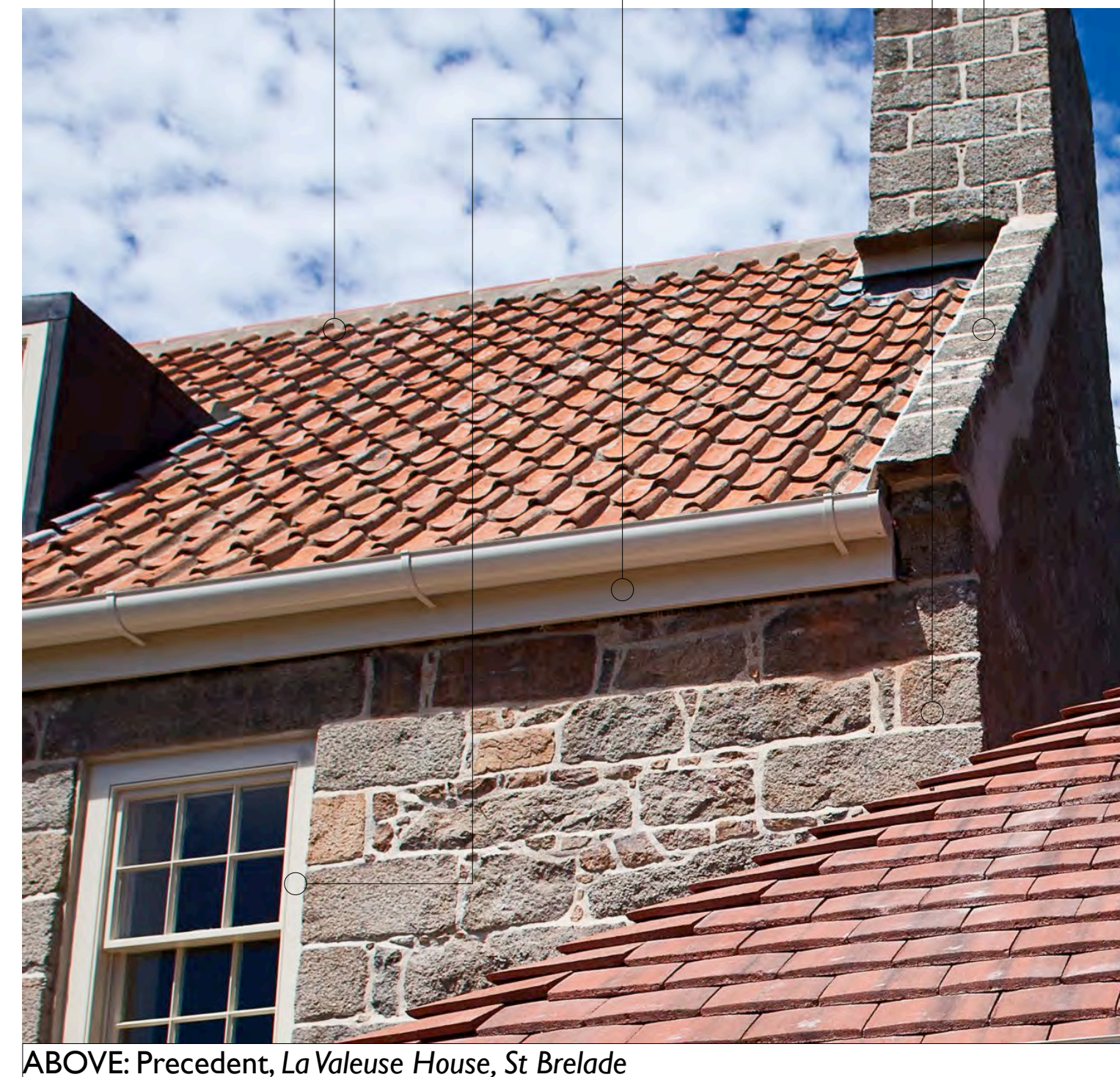
ABOVE: Precedent, La Vaieuse House, St Brelade
