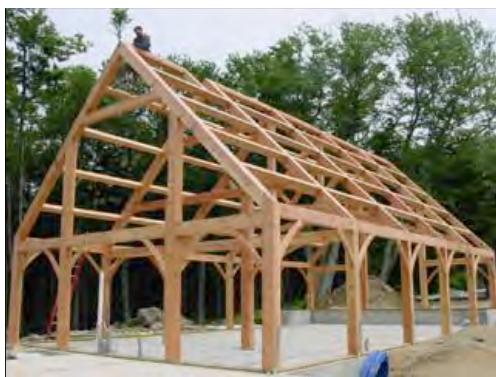
ABOVE: Precedent structure for oak pegged mortise and tenon joinery. With the weight of the structure concentrated on the frame, the interior remains largely open and unobstructed.
