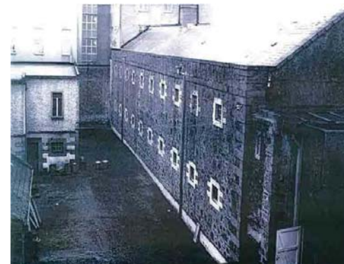
Historic examples of the use of load bearing granite in St Helier.
