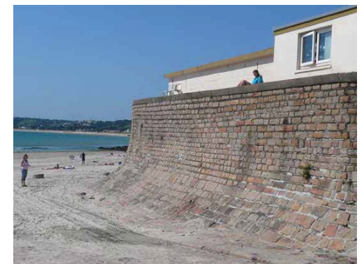
Existing sea wall.
