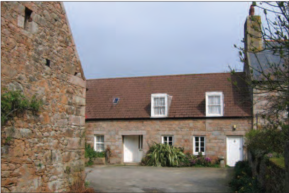
This 17th century single-storey range at Morel, St Lawrence with its cider mill and press (far left bottom), and the wider doorways for cider barrels at Les Ruettes, St John (top), and Hamptonne, St Lawrence (bottom)
