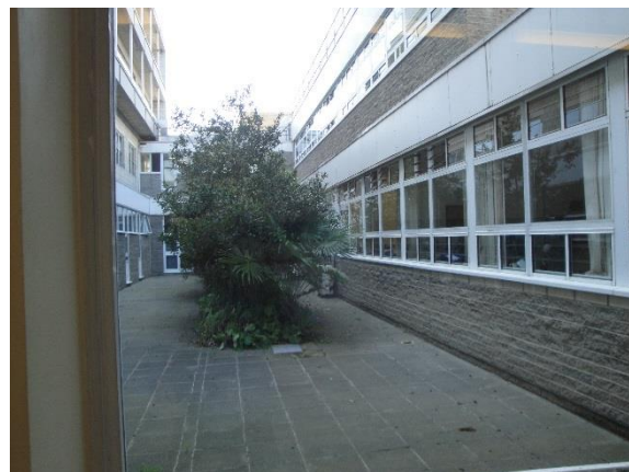
Photograph 1 – Internal courtyard area
