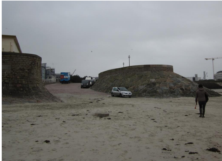
Figure 6 - Wall Type 2 - slipway
