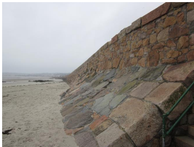
Figure 3 - Wall Type 1 photograph
