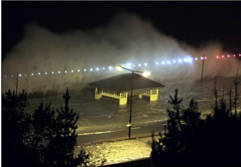
Figure 4 - Overtopped discharge down Victoria Avenue (BBC Jersey)
