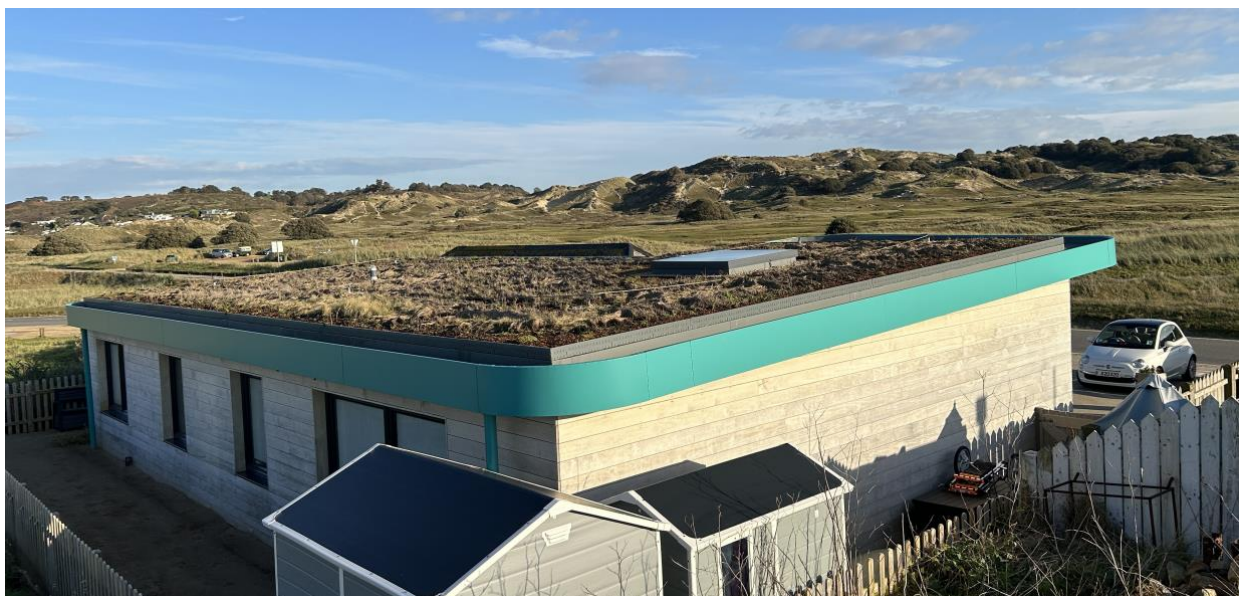
The green roof at Healing Waves, Le Braye, showing how green roofs can soften buildings into the landscape. Red Fescue was used. Photo by Chris Bester
