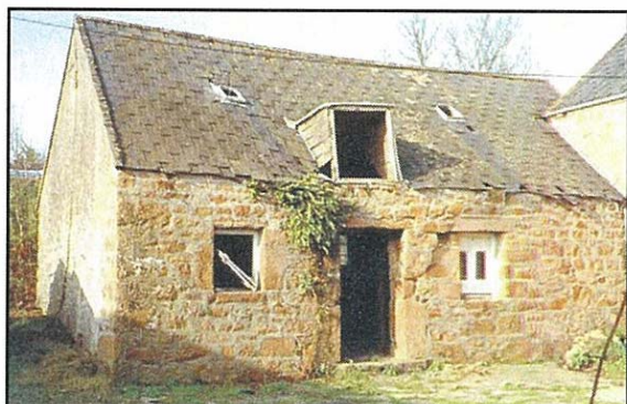
The interior of the Island contains many old farm buildings. These often have a distinctive architectural style arising out of the shortage of timber at the time of construction and the use of the local pink granite
