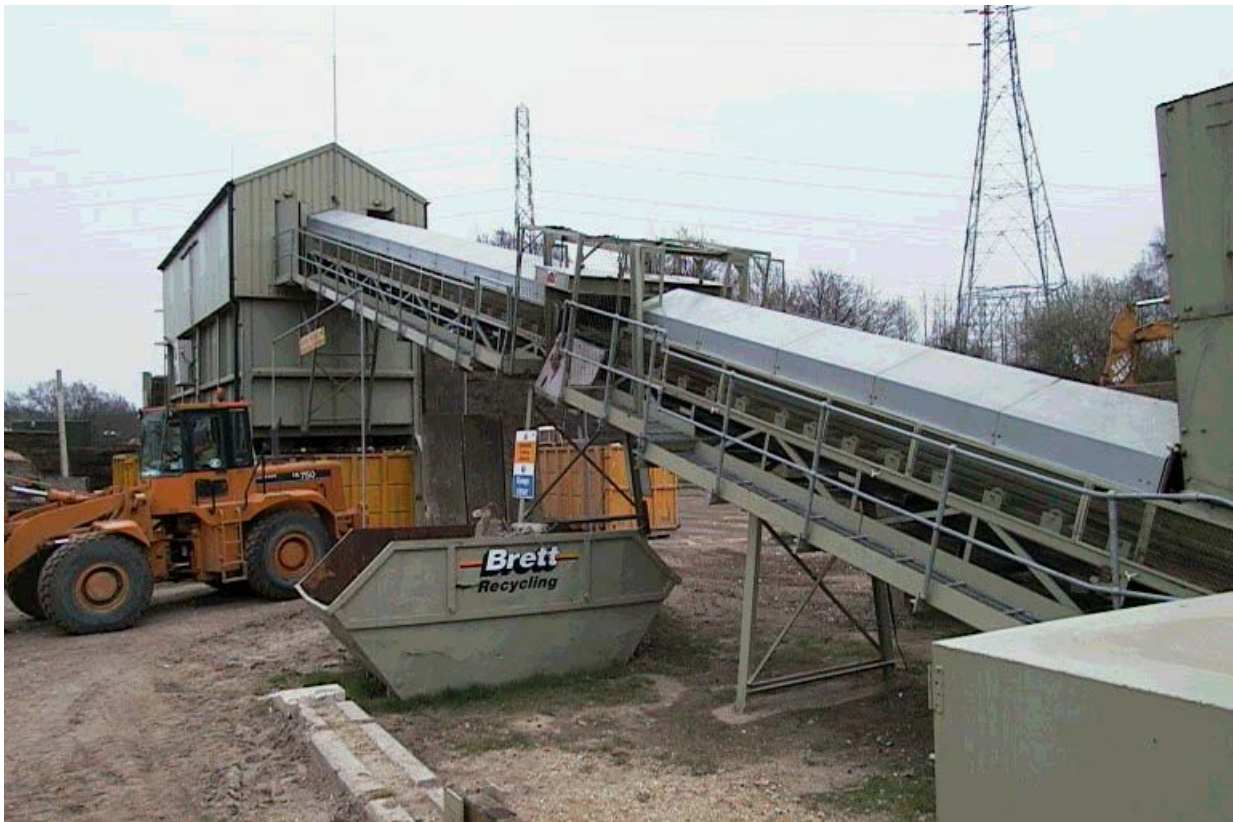
Aggregate Recycling Plant - Shelford Farm Waste Disposal Site, Kent - March 2000
