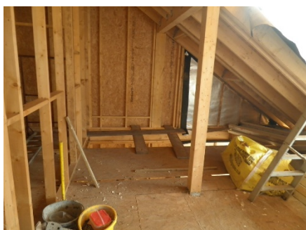
View from first floor
